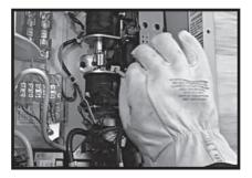
Locate the transfer handle and insert the metal end into the slot in the main contactor assembly. Pull the handle DOWN to move the main contacts to the standby power (generator) position.
